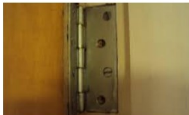
There are less than 3 door hinges or the hinges are missing screws.
